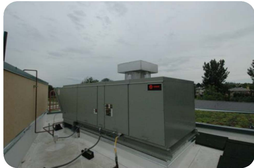
High Efficiency HVAC
